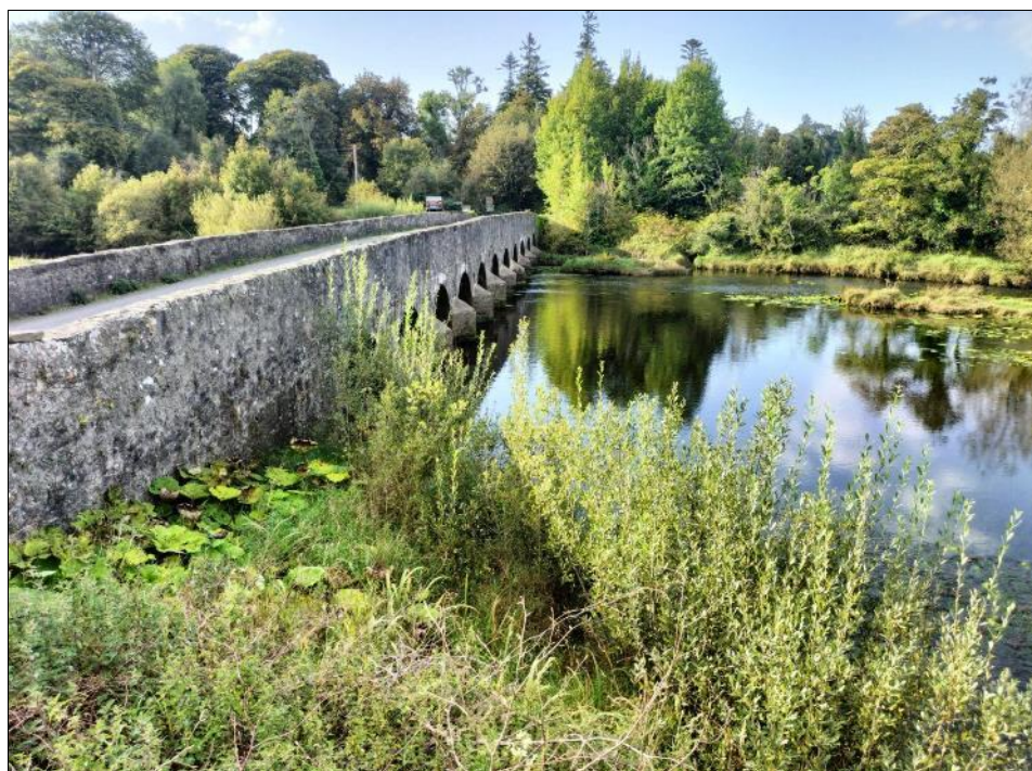
Plate 14.10: View of Palmerstown Bridge
