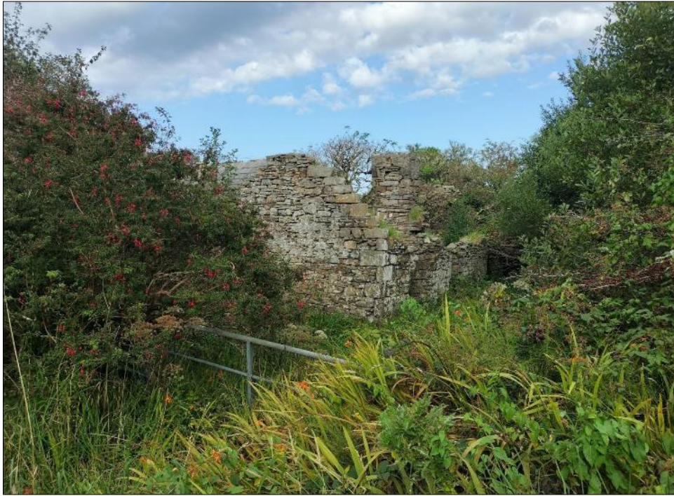
Plate 14.7: View of vernacular structure in Carn townland
